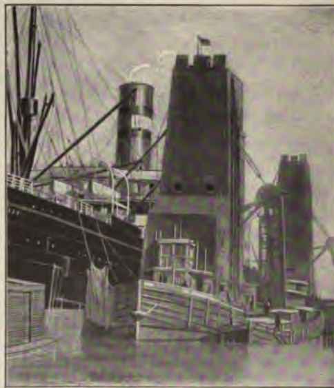
A FLOATING GRAIN ELEVATOR. Transferring grain from a canal boat to an ocean steamer in New York City.
